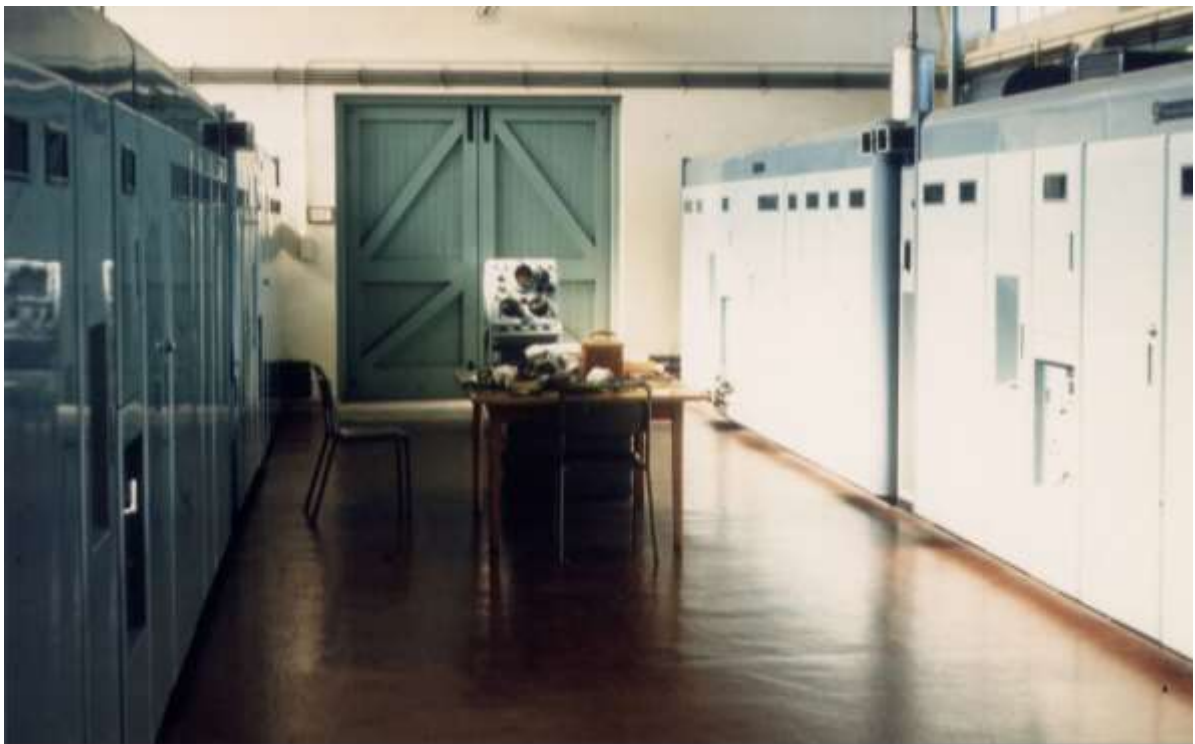
S.T.C. 30kW Transmitters in 'B' Station
